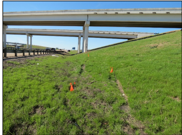
Figure 4: View northwest to area of AE on the embankment
