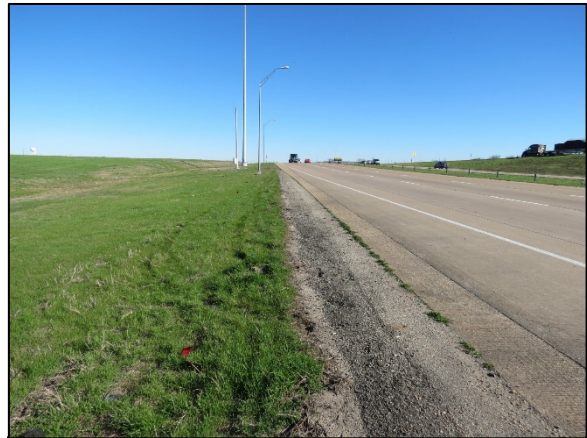
Figure 2: View southeast from the area of roadway departure back to Chevrolet's approach environment
