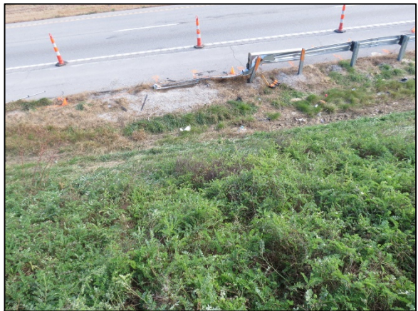
Figure 4. View east to damaged guardrail and final rest position of Mitsubishi.
