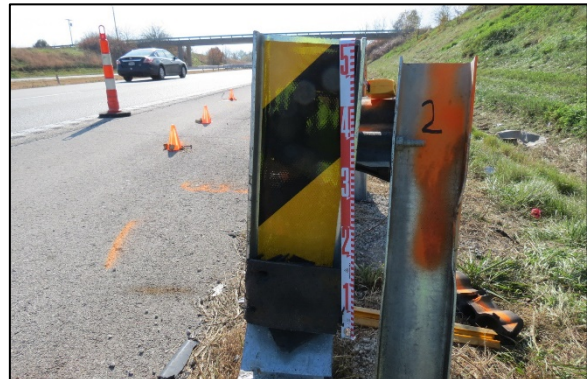
Figure 5. Face of end terminal.
