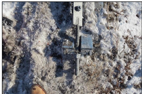
Figure 5: Anchor bolt secured to end of guardrail tab
