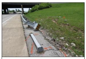
Figure 1. The damaged end terminal and guardrail, view southeast.
