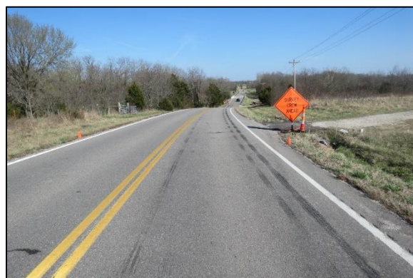
Figure 3: Eastbound approach of the Buick to the area of lane departure
