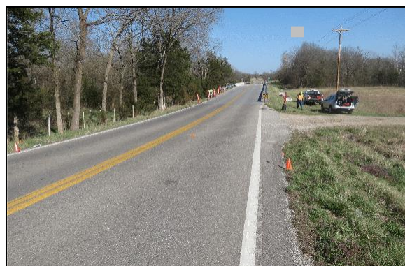
Figure 4: View northeast to area of onset of yaw marks and approach to end terminal impact
