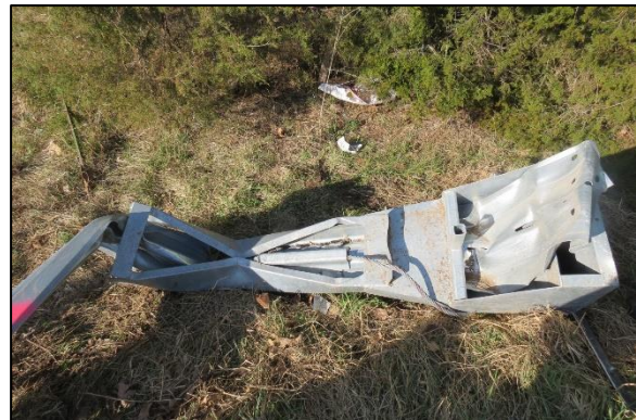
Figure 8: Extruded guardrail and field side of the end terminal
