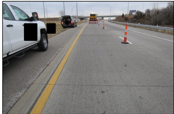
Figure 3. Northwest view of the Ford's approach to guardrail head impact.
