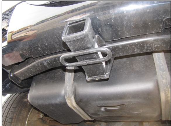
Figure 18: Back undercarriage view of the trailer hitch mounted on an exemplar Jeep Liberty.
