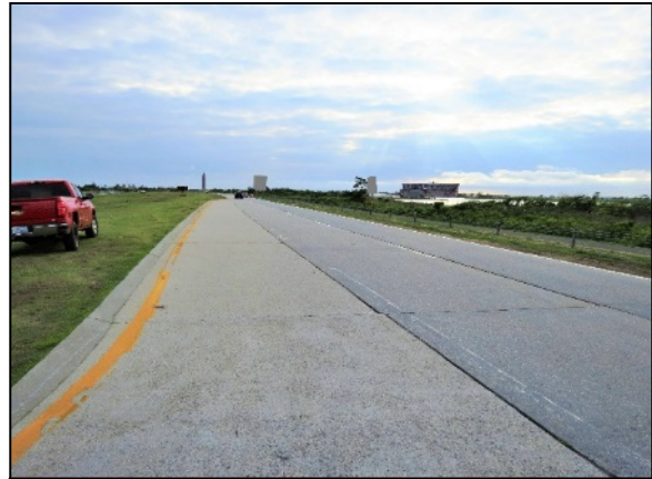
Figure 3. West-facing view of the merge lane and westbound travel lanes.
