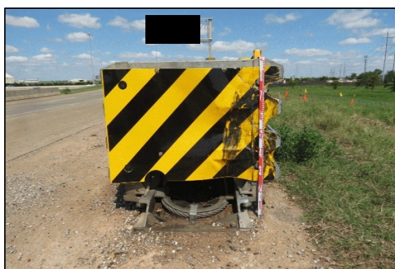
Figure 5. Damage to attenuator from impact by the front plane of the ambulance, view north.
