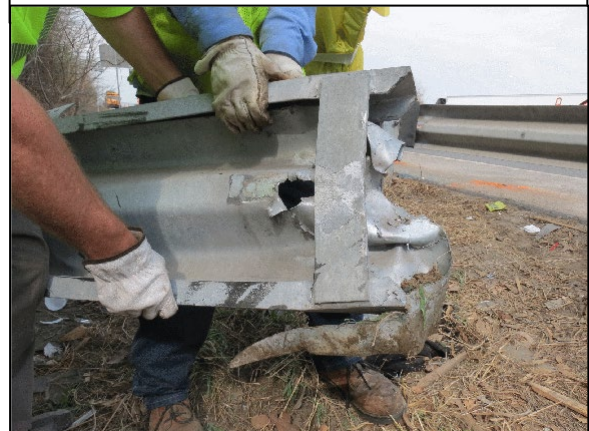
Figure 5. Torn guardrail in feeder channel.
