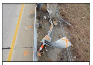
**Figure 5**: ET-Plus and extruded guardrail (west facing lookback view).
