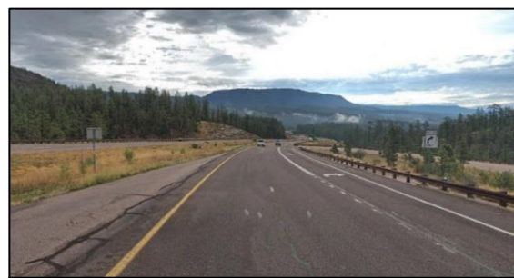
Figure 2. Eastbound approach (Google Maps image).
