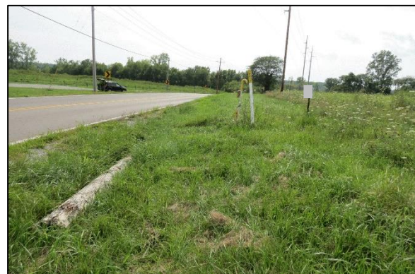
Figure 4: Westerly view of the approach to impact with petroleum pipeline marker post (displaced during impact).
