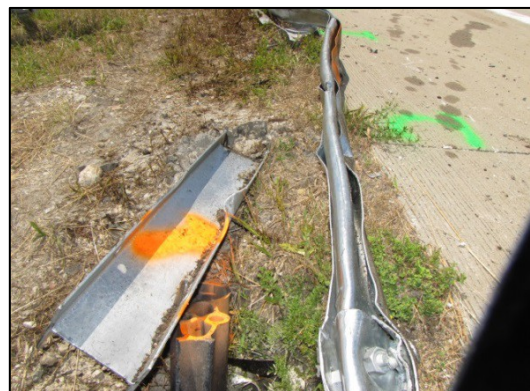
Figure 9. South-facing image depicting the post 2 deformation and the displaced block-out.
