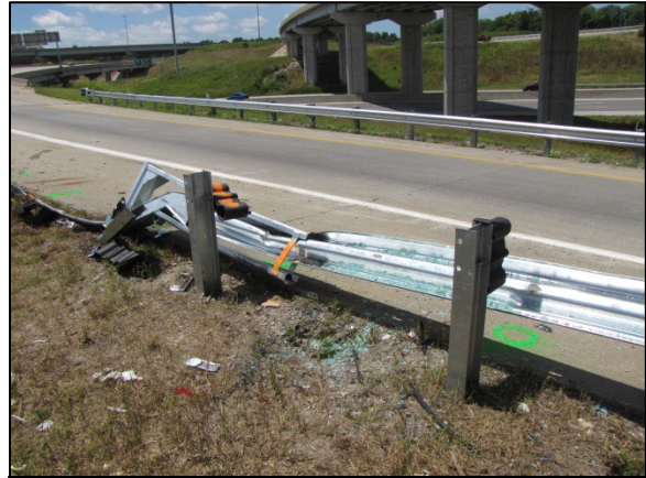
Figure 7. Southwest-facing image depicting the final rest location of the Ford between posts 5 and 6, evidenced by the disintegrated glazing.
