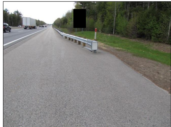
Figure 3. South trajectory view at the crash site and the replaced guardrail system.
