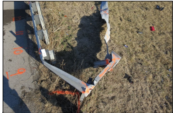
Figure 6. Overhead view of the damaged guardrail and end terminal.
