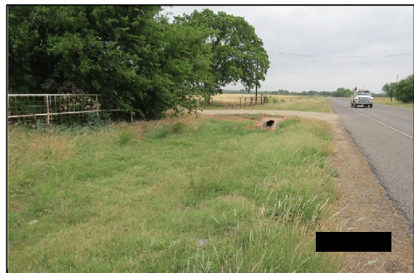
Figure 3. Roadway departure, northwest.
