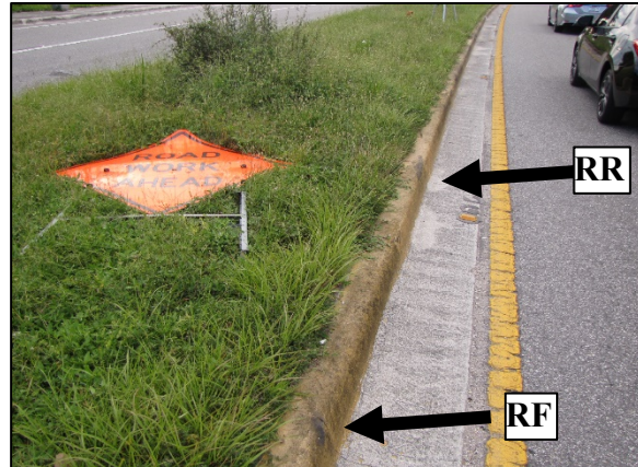
Figure 5. West-facing view depicting the locations of the curb strikes of the Nissan's right front and right rear tires.
