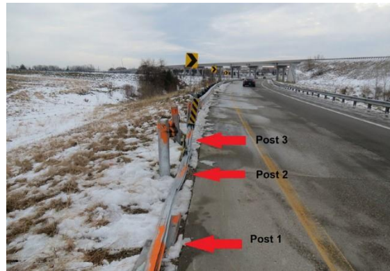
Figure 6. End terminal impact
