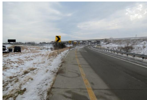
Figure 4. Roadway departure, looking east
