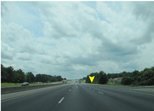
Figure 2. Westbound approach of the Chevrolet; the arrow shows area of roadway departure
