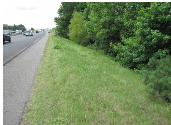
Figure 3. Northwest approach of the Chevrolet down the embankment to the wooded area
