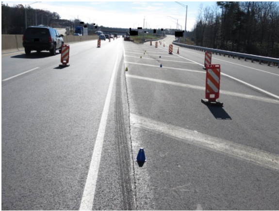
Figure 3. Southbound view of the Kia's departure from the travel lane onto the gore area
