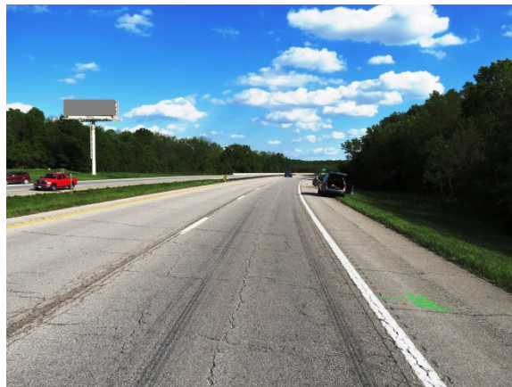
Figure 2. East-facing view of the Nissan's eastbound pre-crash travel trajectory on the divided roadway
