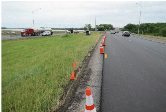
Figure 4. Location where the Chevrolet departed the roadway and entered the median, small orange cones shows path of left side tires
