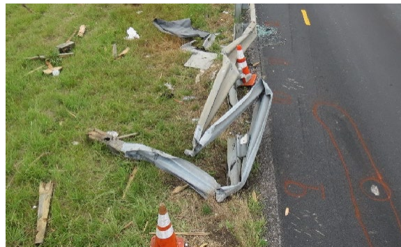
Figure 11. Kinks in the damaged guardrail
