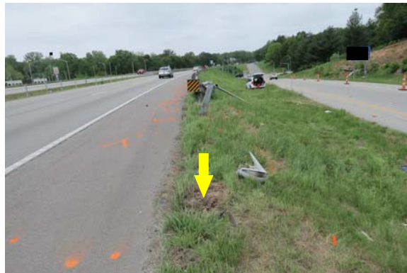
Figure 3. Southwest view, impact with luminaire
