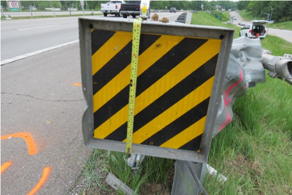
Figure 5. Southerly view, head of end terminal
