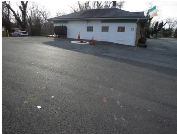
Figure 4. West-facing view of the Toyota's rotating tire marks (paint highlights) en route to impact with the bollards and the building
