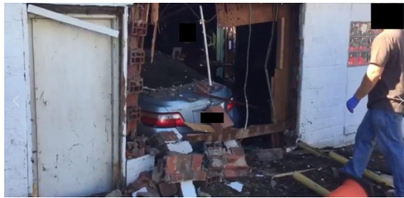
Figure 1. East-facing view of the Toyota at final rest in the commercial building. (Image obtained from an internet news source)
