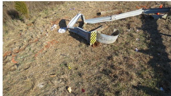
Figure 2. The damaged guardrail and guardrail head, view east
