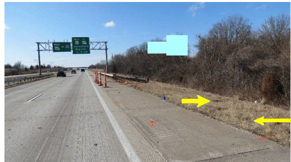
Figure 5. Approach of the Pontiac to impact with the guardrail head, arrows show yaw tire marks on shoulder, view northwest
