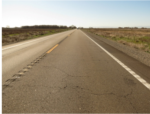
Figure 2. Approach to crash site looking south
