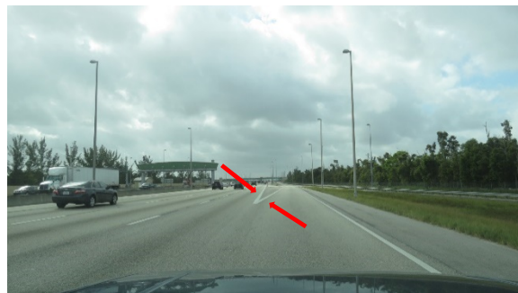
Figure 3. Southbound view of the original travel lane and the exit travel lane lines where they meet
