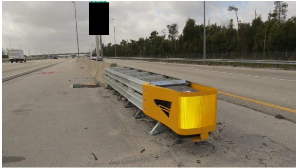
Figure 4. QuadGuard II impact attenuator system
