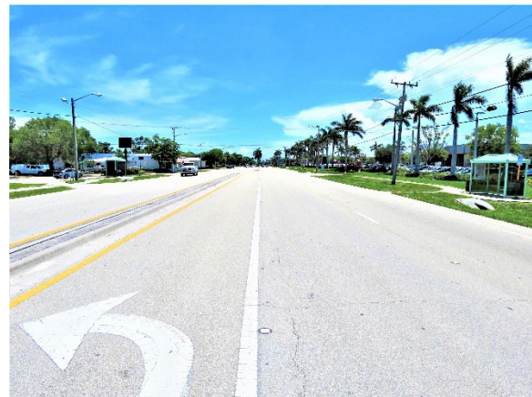
Figure 3. South-facing view of the southbound travel lanes and left turn lane on approach to the intersection
