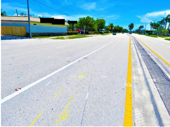
Figure 5. South-facing view of the northbound lanes and crash trajectory evidence (yellow and white markings within the travel lanes)
