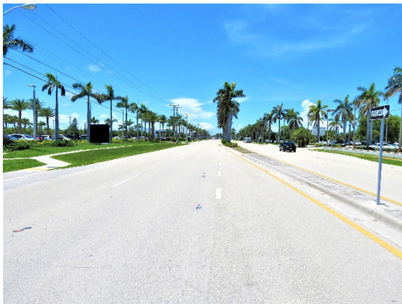
Figure 2. North-facing lookback view of the southbound travel lanes
