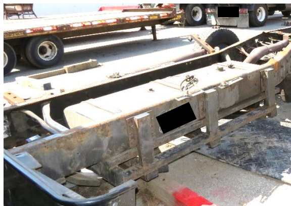
Figure 13. Right oblique view of the bus's fuel tank and surrounding safety cage
