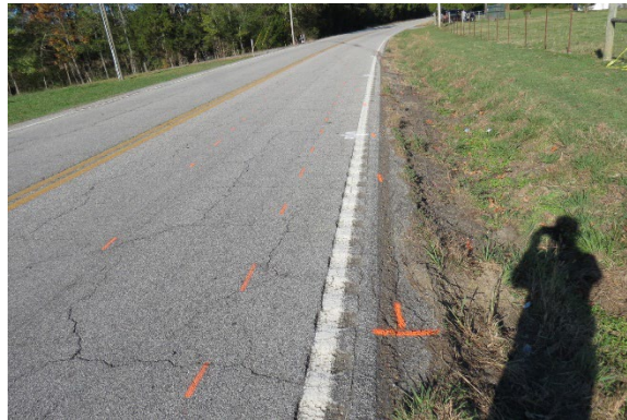
Figure 4. North view of the Freightliner's pre-crash travel path
