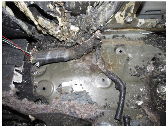
Figure 14. View after the removal of the fire debris at the base of the Infiniti's B-pillar
