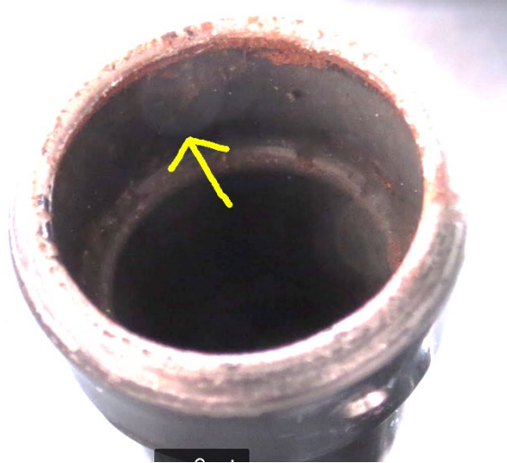
Figure 16. Interior top (no peening markings)
