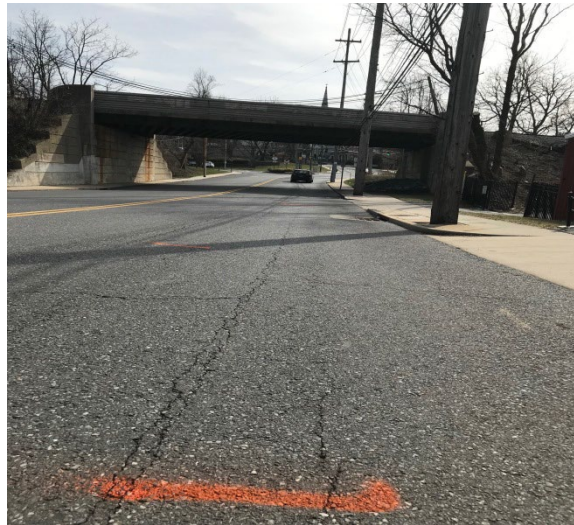
Figure 4. Police image of the Nissan's eastbound approach to the crash site
