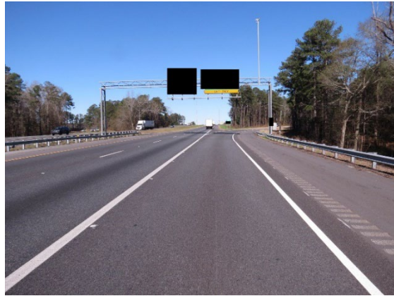
Figure 2. Viewing north along the Ford's approach
