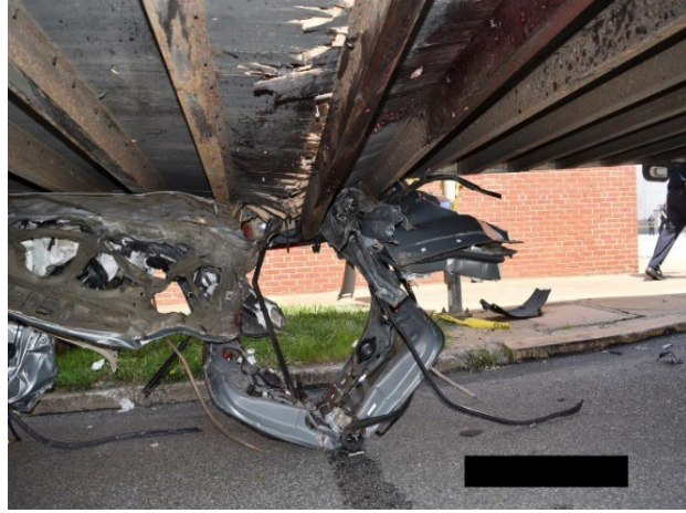
Figure 21. Trailer exterior damage looking from the left plane (On-scene police image)
