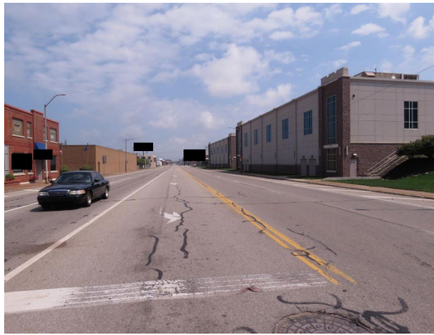
Figure 3. Viewing east of the crash scene, looking back
