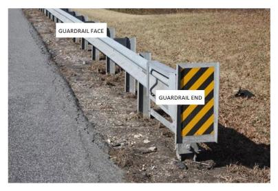
Figure 1. Guardrail face and guardrail end. Source: FHWA
