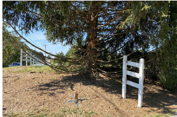
Figure 7. View of the Event 5 (fence) and Event 6 (tree) area during the SCI scene inspection
