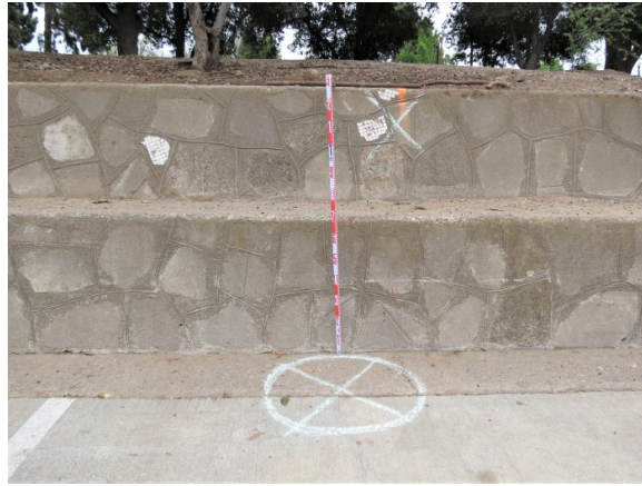
Figure 4. Stone wall looking south, area of crash events 3 and 4
