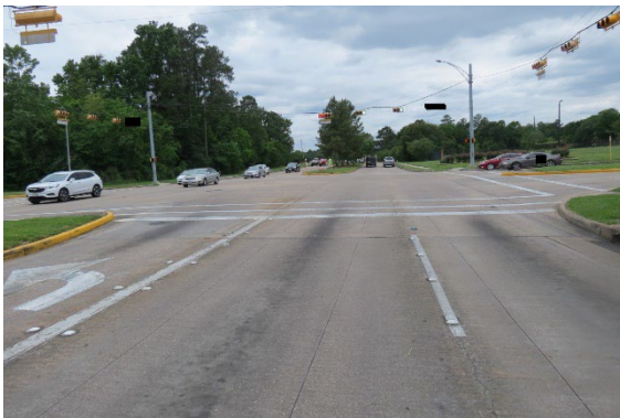
Figure 2. West view of the ambulance's approach
