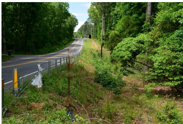
Figure 4. Facing north at the sections of the cable barriers
