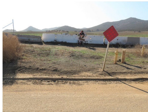
Figure 4. Crash site, area of end departure and concrete traffic barrier, looking south
